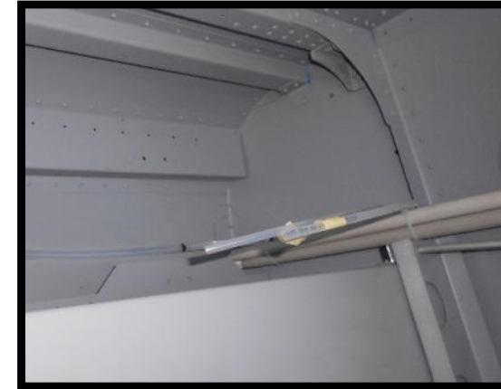
Pipes under front platform left Tubi sotto pedana anteriore SX
